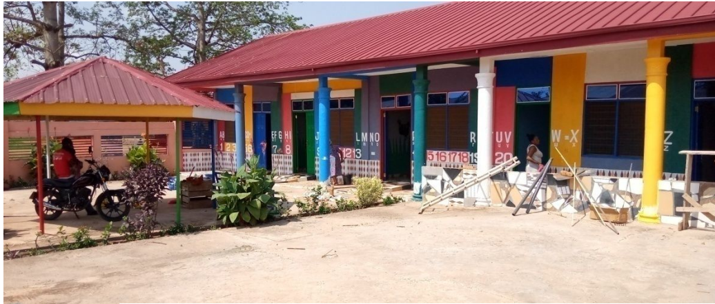
Figure 15: The new daycare center at Nkoranza
