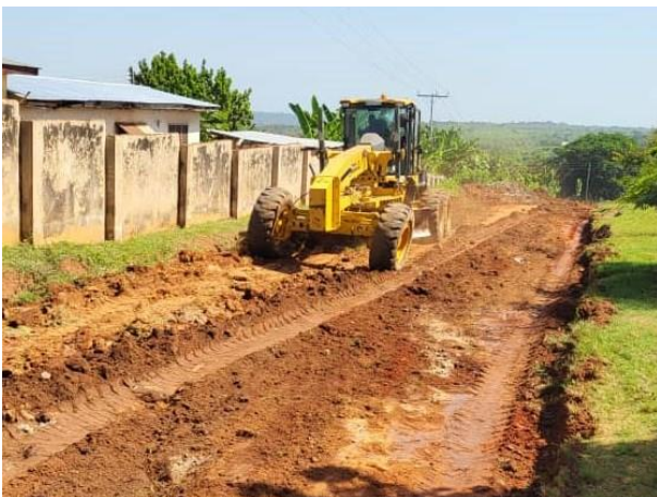
The new road (by then under construction)
