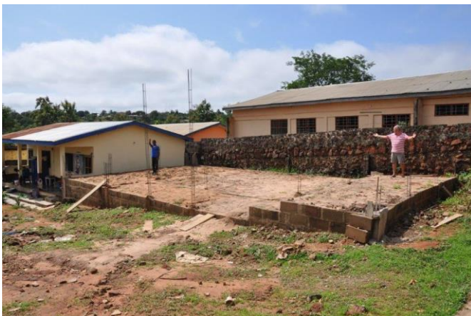
The foundation of the new and bigger Boys Dormitory,
